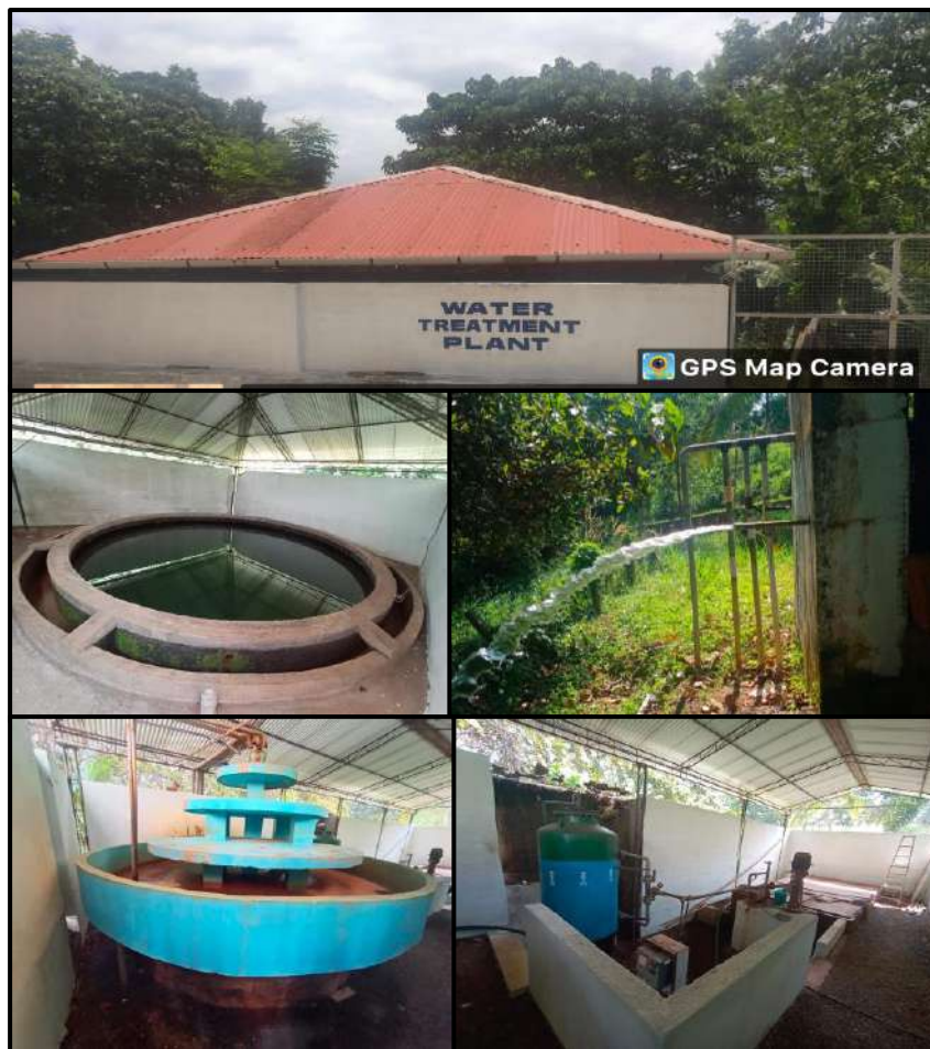
Water Treatment Facilities in the College Campus
