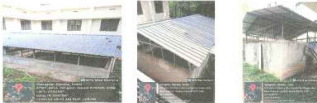
Figure 1: Rainwater harvesting tank
