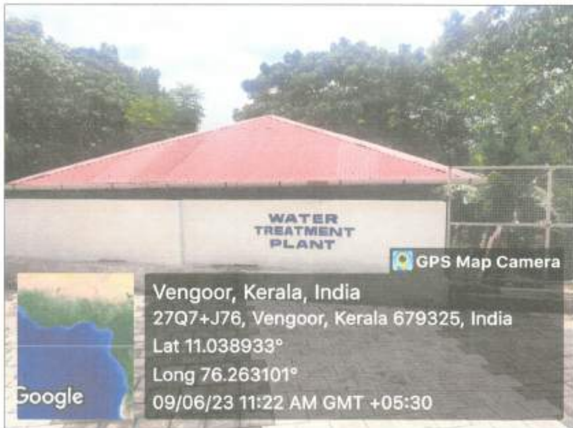
Waste Water treatment plant.
